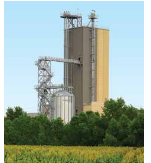
ASI-Industrial, the subcontractor responsible for building the slip-formed concrete main tower, also approved and installed all the equipment in the facility. ASI specified Baldor products almost exclusively on its projects and was not surprised that other OEMs participating were also choosing Baldor.
